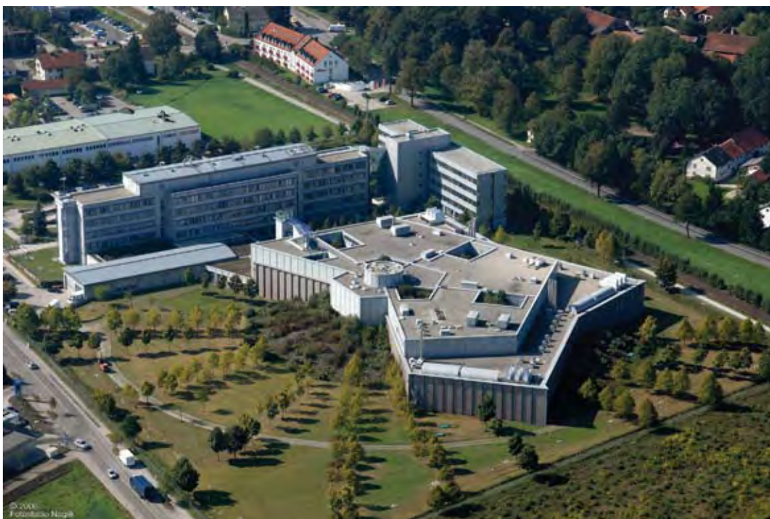
Amadeus Data Centre, Erding, Germany
